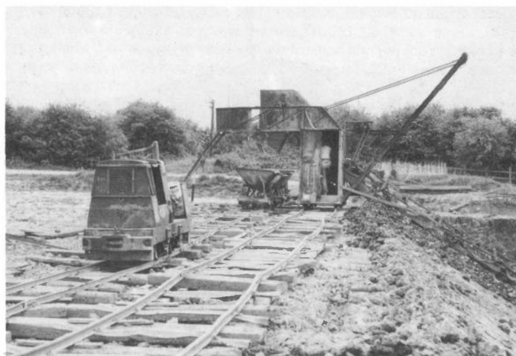
Ruston 223692 arrives at the tipping shed with four full wagons whilst the empties stand on the left awaiting the return journey to the clay pit. (A.J. Booth)
